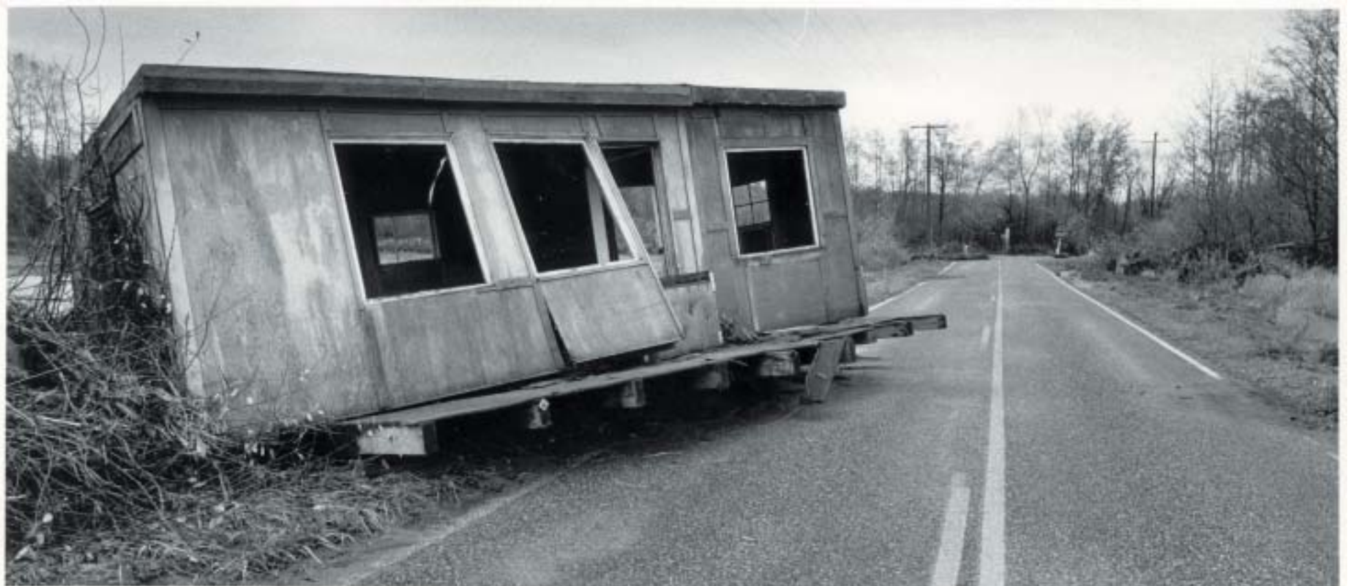
Debris from the November 1990 flood lies across Ferndale Road. (Photo: courtesy of the Bellingham Herald)
