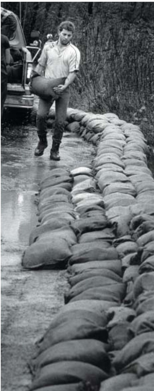
Sandbags can provide temporary protection from floods. During a flood emergency, county residents can request sandbags by calling (360) 676-6681. (Photo: courtesy of the Bellingham Herald)
