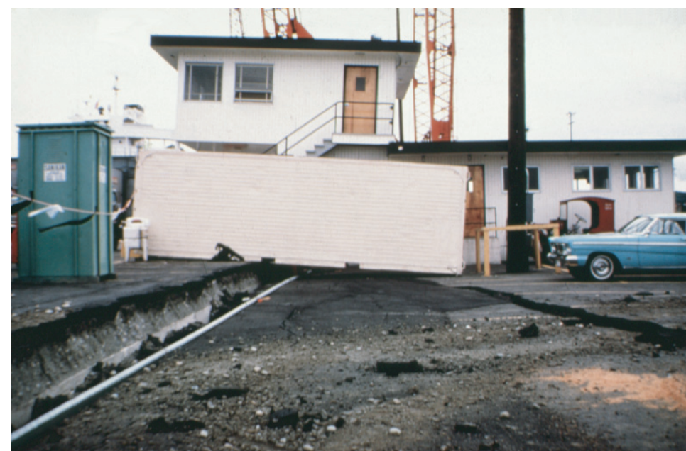
Liquefaction during the 1965 SeaTac earthquake caused both lateral and vertical movement of the ground in the Port of Seattle. Cargo cranes such as the one in the background are vulnerable to liquefaction-induced ground displacement. Lateral spreading such as this can cause severe damage to both above-ground structures and underground utilities. Photo courtesy of the Karl V. Steinbrugge Collection, Earthquake Engineering Research Center ( http://nisee.berkeley.edu/visual_resources/steinbrugge_collection.html ).
