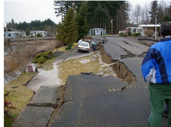
Liquefaction: 2001 Nisqually Earthquake
